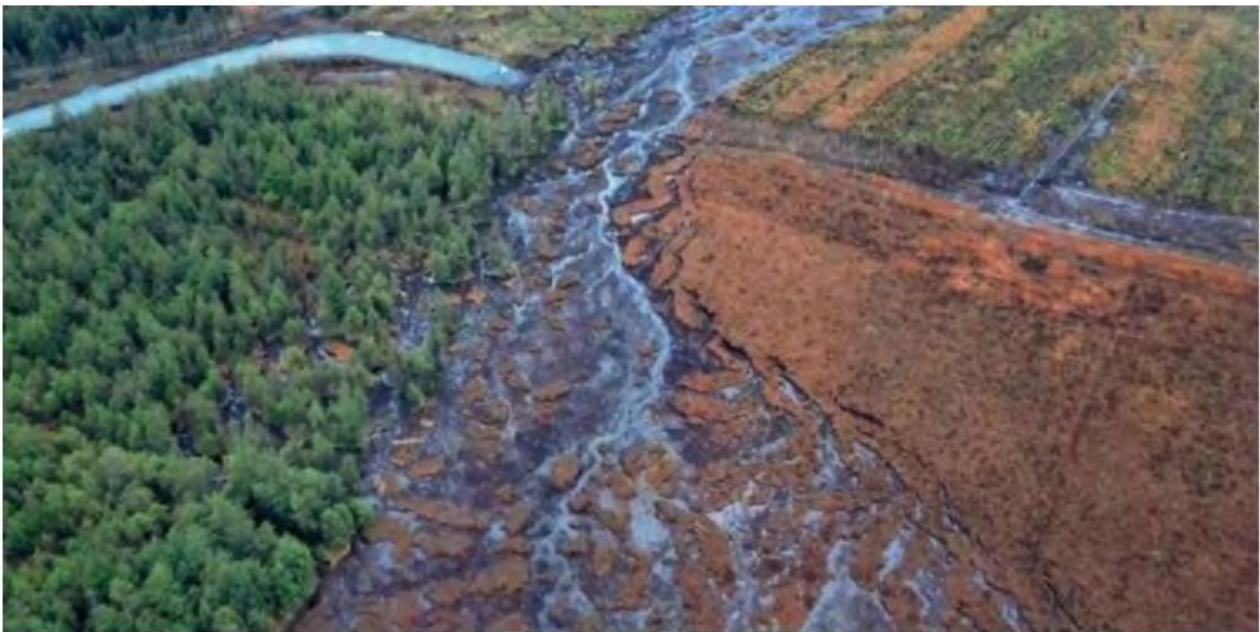
Plate D Previously concluded 'No Potential for Impact' Meenbog Wind Farm site, which failed in in 2020. (photo credit Donegal Live 4 th January 2024).
