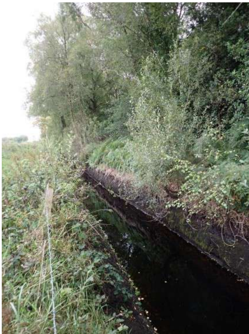
Fig. 25: Typical Existing Drain Cut into Peat at the Site (Source: Appendix 8-2 Peat Stability Risk Assessment, Figure 7)
