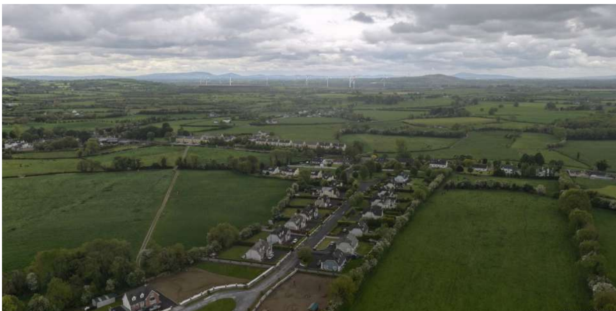
Figure 8-43: Riverstown and view of Turbines
